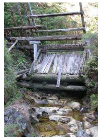
Above: Lower Kaiaraara dam Photo in 2009. View looking upstream.
