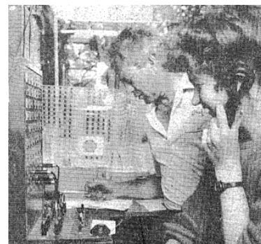
Old Telephone exchange Tryphena 1985
