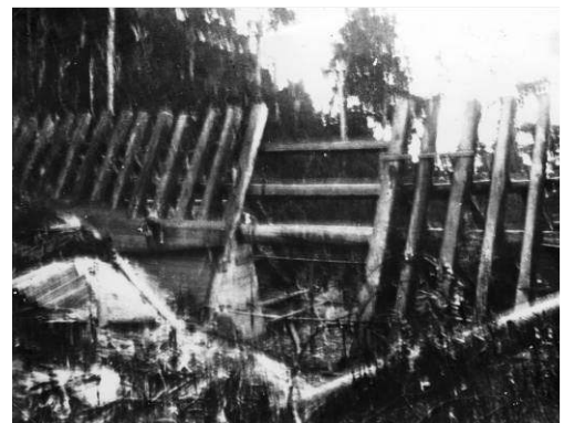
Lower Kaiaraara dam in construction 1924. View from upstream looking down
